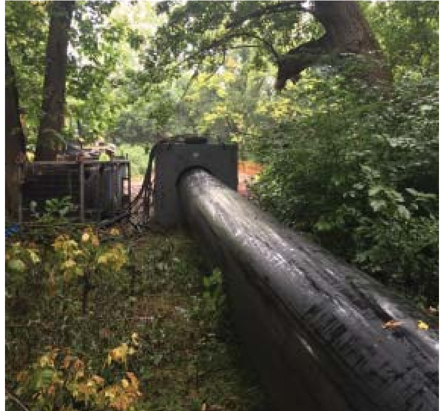
Pipe being pulled and compressed through roller box
