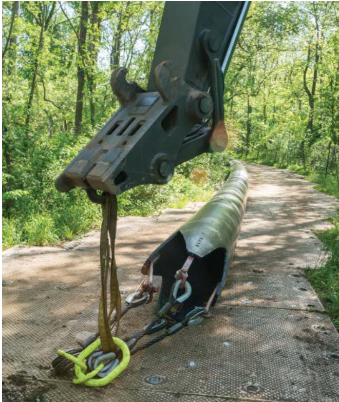
Pipe being pulled and compressed through roller box
