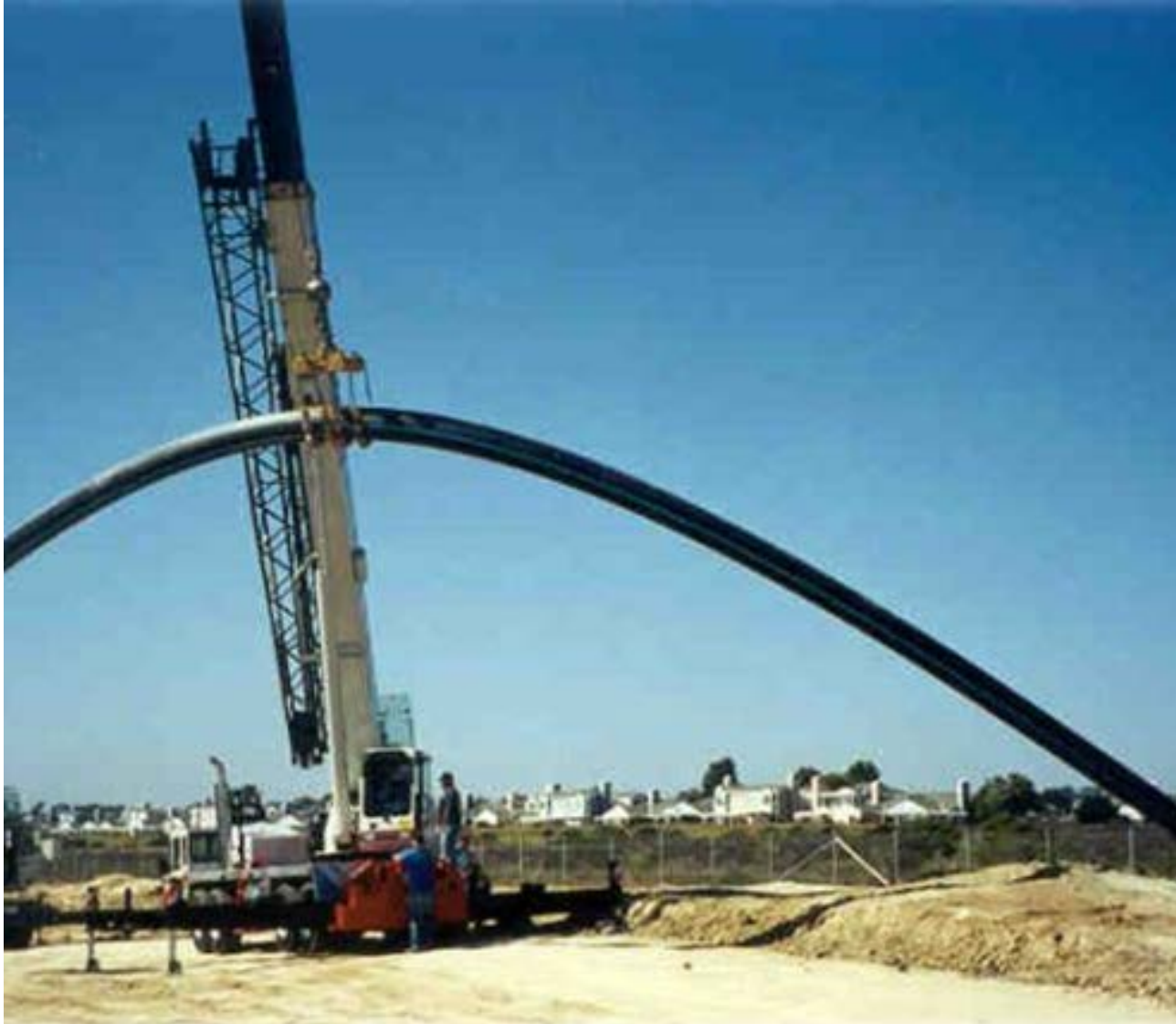
20" installed under I-5 California
